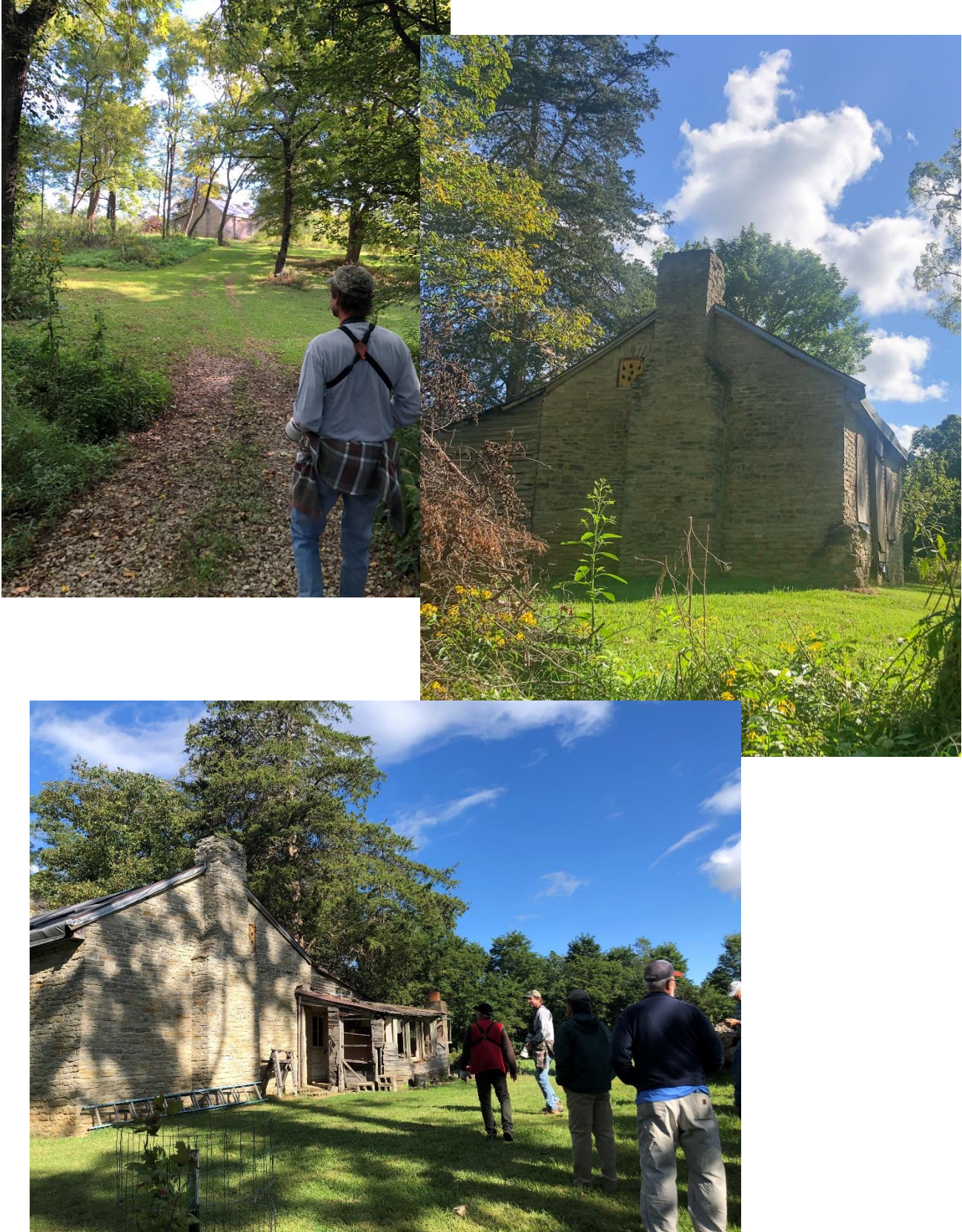
Hultz stone house- constructed 1831, currently under restoration. Pics by Harriet Moore
